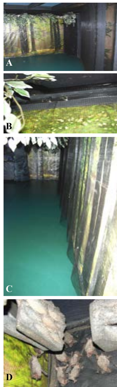
Figure 6-7. A: Solid and open flight enclosure walls meet in the corner. Mesh attached to open framework is secured tightly against the frame with staples, leaving no gaps in which bats can escape. B: A mesh panel attached to steel binding with magnets. C: Mesh panels provide a cushioned landing and are easily removed for cleaning. D: Free-tailed bats that have chosen to roost behind mesh, allowing easy inspection of body condition. T. brasiliensis . Bat World facility. Photos by A. Lollar.
