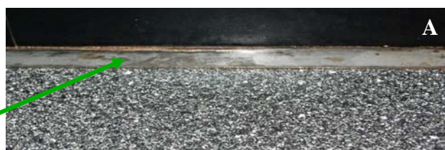
Figure 6-10. A: A laminated floor can be easily cleaned with a whisk broom. Flat metal binding is used to seal the edges of laminate.
