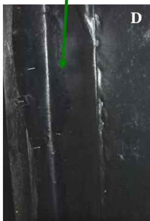
Figure 6-10. D: The outer door frame edge covered in vinyl to prevent bats from gaining a foothold and roosting in the hinged area of the door where they may become crushed. Bat World facility. Graphic by L. Crittenden.
