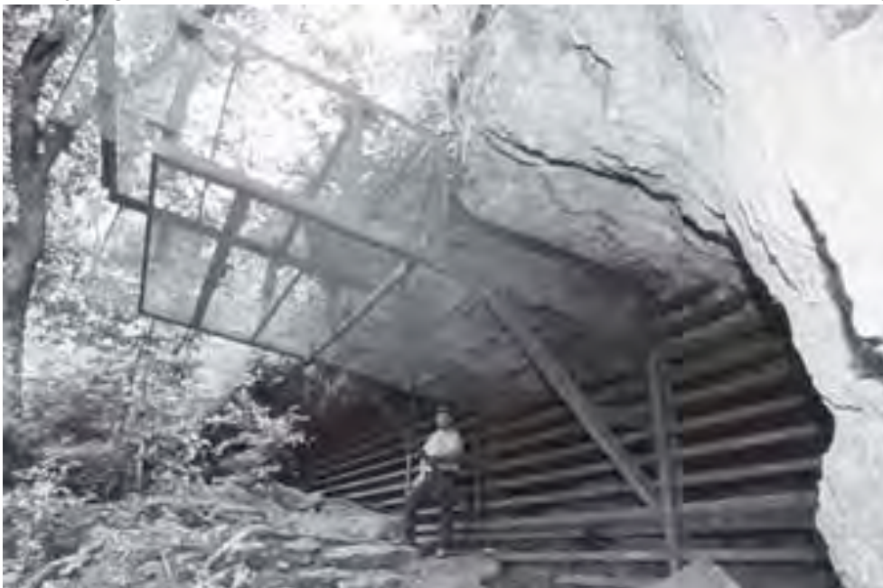
Figure 5. Chute gate at McDowell Cave, Missouri © 2001 Sheryl Ducummon
