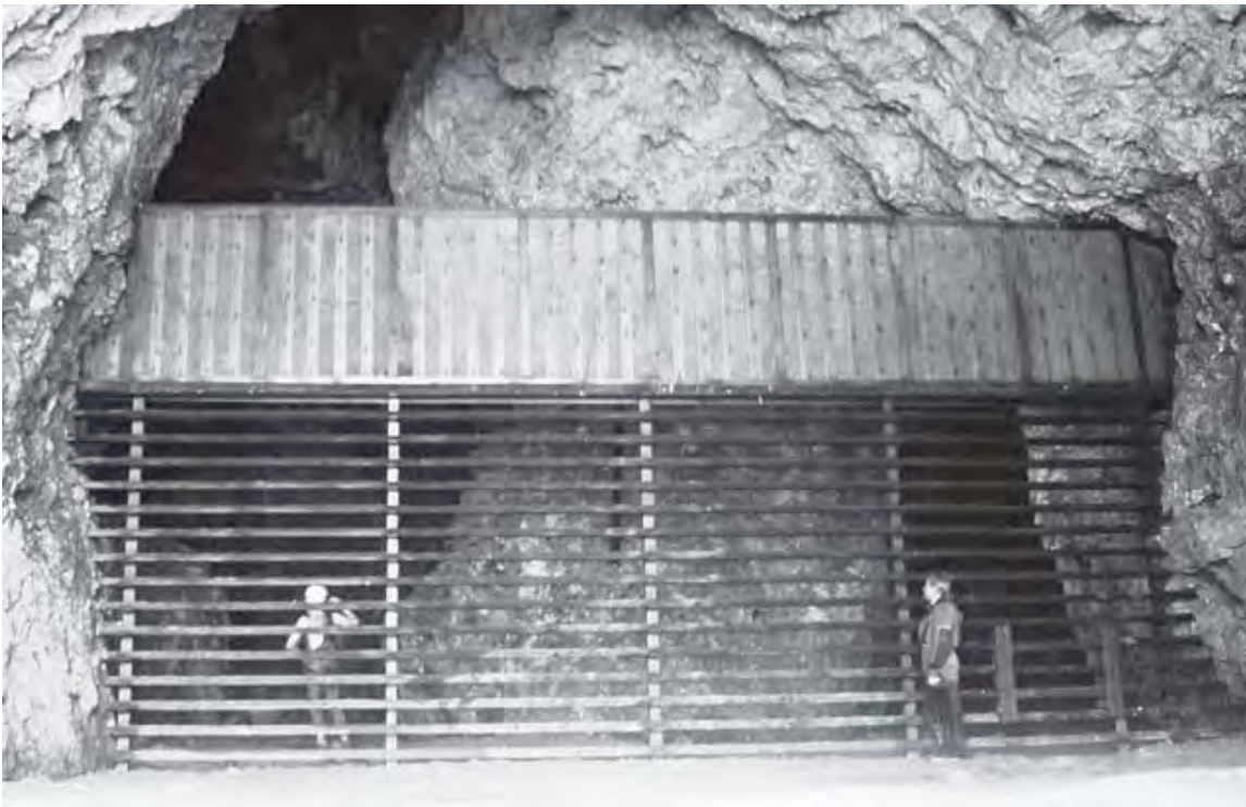
Figure 9. Half or “flyover” gate. Note the removable bar at bottom right. Expanded metal mesh covers the overhanging top portion, making it extremely difficult to climb over. Coating the overhang with grease also helps repel trespassers. © 1997 Keith Christenson, BCI
