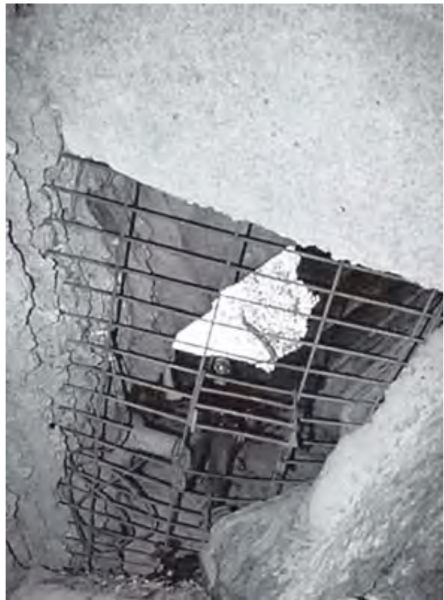
Figure 2. This is a poorly designed gate, constructed of 1-inch (25-millimeter) round bars. It is not very secure—the bars maybe easily bent and the welds are small. The small rectangular openings in the narrow vertical entrance make the gate difficult for bats to fly through. On this type of platform gate constructed in a vertical entrance, branches and leaves can collect to restrict airflow and light. © 1989 Jim Kennedy, BCI
