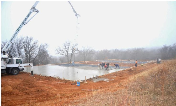
**Left:** In January of 2014 a 60 foot by 120 foot concrete foundation was poured.
