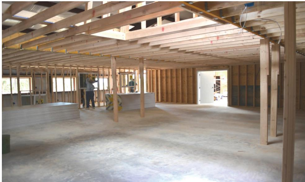
**Above:** Framing of the inside flight enclosures was near complete in May, which then allowed the stainless steel framework for the interior cage to go up. The windows shown in the background lead to the office area (page 35), and the double doors lead to the semi-outdoor flight cage (page 33).
